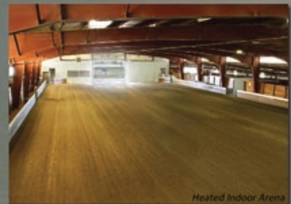
Heated Indoor Arena
